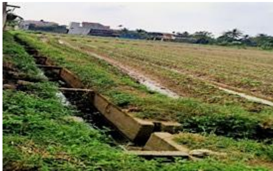
In-field irrigation canal
